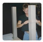
Step 2: Slide base trim onto posts. Locate bottom bracket position by measuring 3/4" from top of base trim, using a pencil, draw a line.
