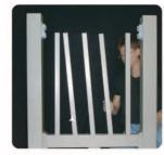
Step 10: Starting at one end begin inserting spindles into holes in bottom rail.
