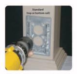
Step 5: Attach bottom bracket plate to posts using 6 - 2" stainless steel screws (provided) per bracket. Position bracket plate as shown.
