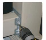
Step 9: Secure rail to brackets by attaching 4 - 1" stainless steel screws (provided) per bracket. Pre-drill holes for easier application. IMPORTANT: Skipping this step will void the warranty.
