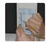
Step 3: Place bottom edge of bracket plate on line, center on post and mark screw
