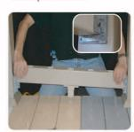
Step 8: Place bottom rail onto bracket plates making sure rail rests firmly on tabs as shown.
