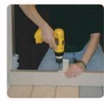
Step 7: Attach center support to center of bottom rail using screws provided. Drill (2) 3/8" weep holes. **IMPORTANT:** Slide trim pieces onto both ends of bottom rail
