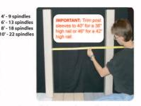
Step 1: Slide on post sleeves. For Standard and T-Rail only, measure distance between sleeves and, if needed, make any adjustments to rail length. Subtract 1/4" from measurement trimming rails and H-channel equally on both ends. NOTE: Remove H-channel prior to cutting rail and then reinsert. If installing contoured or custom railing sections, no adjustments are necessary.
