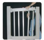
Step 11: Slide trim pieces onto both ends of top rail and begin feeding the rail down onto the pickets. Make sure rail is resting firmly on tabs as shown. Repeat Step 9 for securing rail. Place a small bead of vinyl adhesive to the tabs on inside of trim pieces and press firmly into place.
