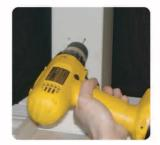
Step 4: Pre-drill marked holes for easier application using a 1/8" drill bit.
