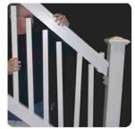
Step 9: Slide trim pieces onto both ends of the top rail. With spindles in place reposition top rail by feeding rail down onto spindles. Repeat Step 6 for securing rail to bracket.
