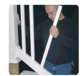
Step 7: Starting at one end, begin inserting spindles into holes in bottom rail.
