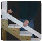
Step 1: Lay the bottom rail as close to the stair treads as possible and up against the posts. While maintaining a 33° angle, and making sure to keep the spacing between the spindle hole and the post the same on top and bottom clamp rail to post.
