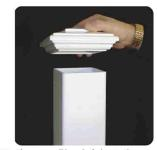
Step 10: Place a small bead of glue to the inside rim of the cap and set onto post.
