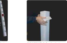
IMPORTANT: Before beginning, make sure all posts are plumb. If using post base trim, be sure to install prior to railing installation. We recommend using a 48" post at the end of the stair run.
