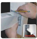
Step 4: Keeping bottom rail as close to stair treads as possible and maintaining the 33° angle, slide the bracket into position making sure that the bottom edge of the rail is resting on the base plate lip. Mark the position of the base plate and remove bottom rail.
