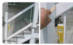
Step 2: Place a spindle in the first and last hole, set top rail and plumb spindles. Clamp top rail to post, using a pencil draw miter lines on top and bottom rail.
